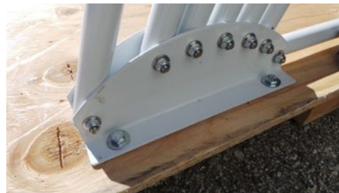
Secure game to plywood using 1.5" bolts, washers, and nuts
