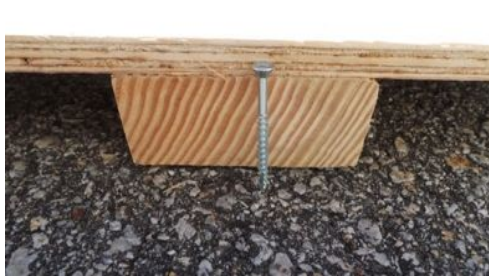
Attach 2x4s to plywood using 2" screws
