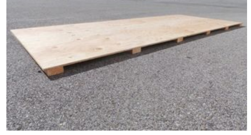
Finished base - for best results apply a standard patio or deck waterproofing agent / sealer
