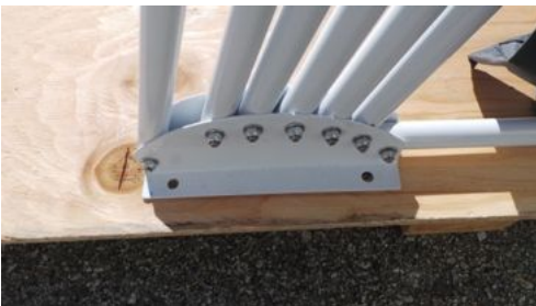
Locate two anchor holes on both sides of frame assembly. Mark and drill holes.
