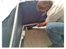
13. Fit the shelter by pulling the cover down around the corners.
